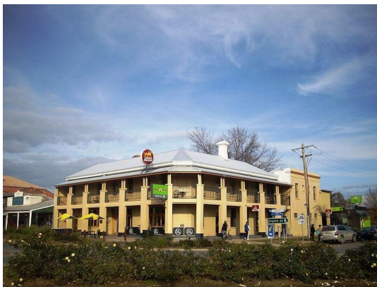
The Mansfield Hotel Where a fire started in the kitchen.
