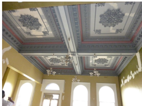
Example of heritage project with interior decorative finishes using “passive fire protection coatings”
